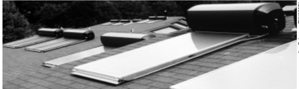
Thermosiphon solar water heaters on employee housing at Yosemite National Park
