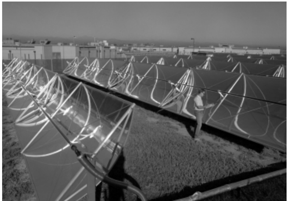
Fig. 10. Parabolic trough solar water heating system for Adams County, Colorado, Correctional Facility.
