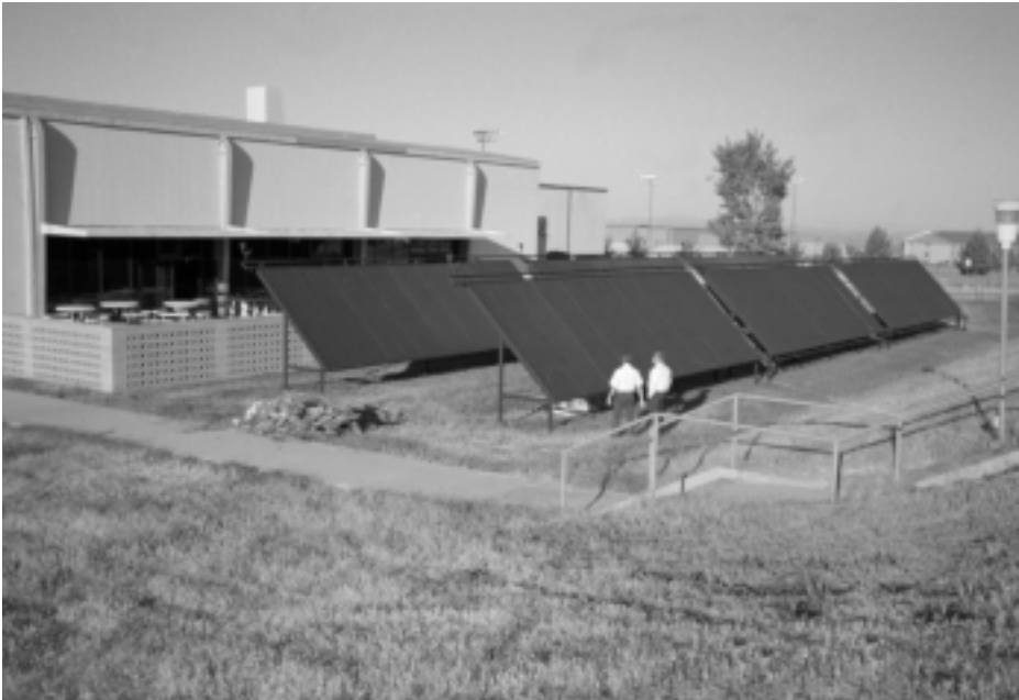
Fig. 11. Solar water heating system for indoor pool at Barnes Field House, Fort Huachaca Army Base.
