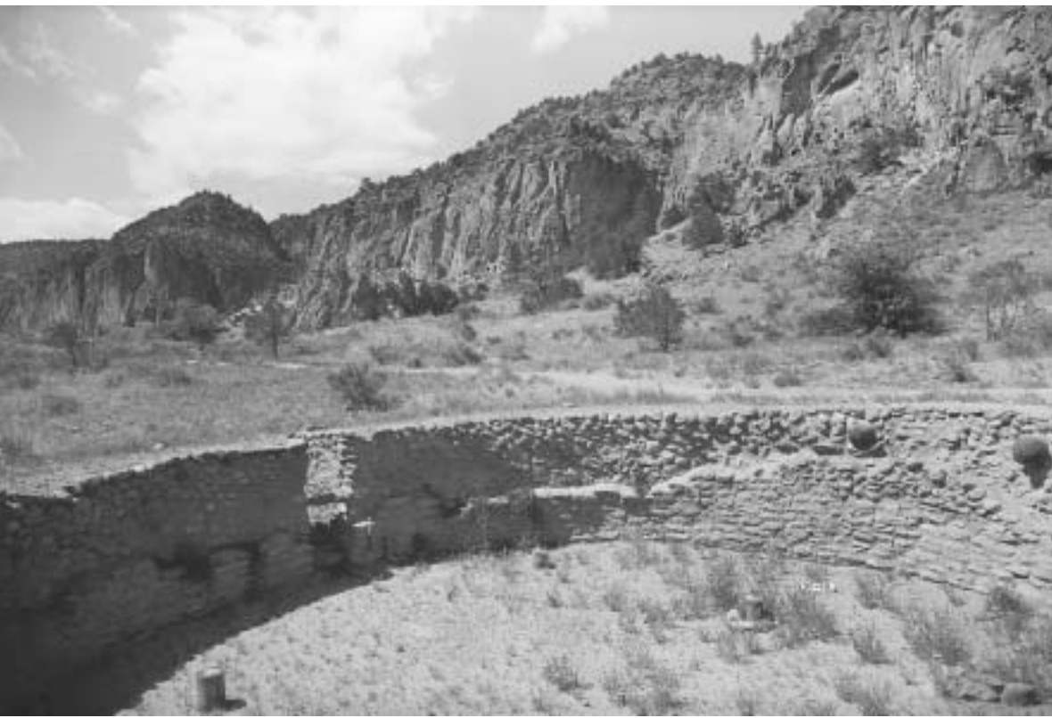
Above: Kiva, vicinity Bland, New Mexico, Donald W. Dickensheets, photographer, 1940; Right: Prudhomme-Hughes Building, Natchitoches, Louisiana, Lester Jones, photographer, 1940
