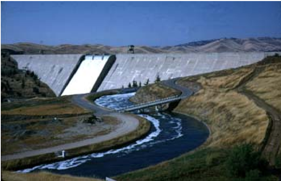
Figure 2 - Friant Dam downstream face.
