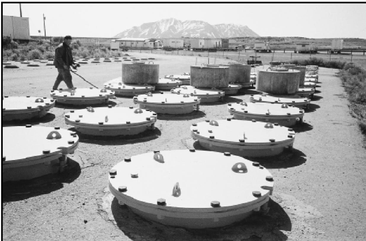
Transuranic waste storage. A radiological control technician scans the ground for contamination at a transuranic waste storage facility in Idaho. Beneath each concrete plug is a vault for storing three or four drums of remote handled transuranic waste. Most of the vaults are currently empty. Waste stored in these vaults is mostly from nonweapons research at the nearby Argonne National Laboratory-West. Intermediate Level Transuranic Waste Storage Facility, Radioactive Waste Management Complex, Idaho National Engineering Laboratory, Idaho. March 17, 1994.
