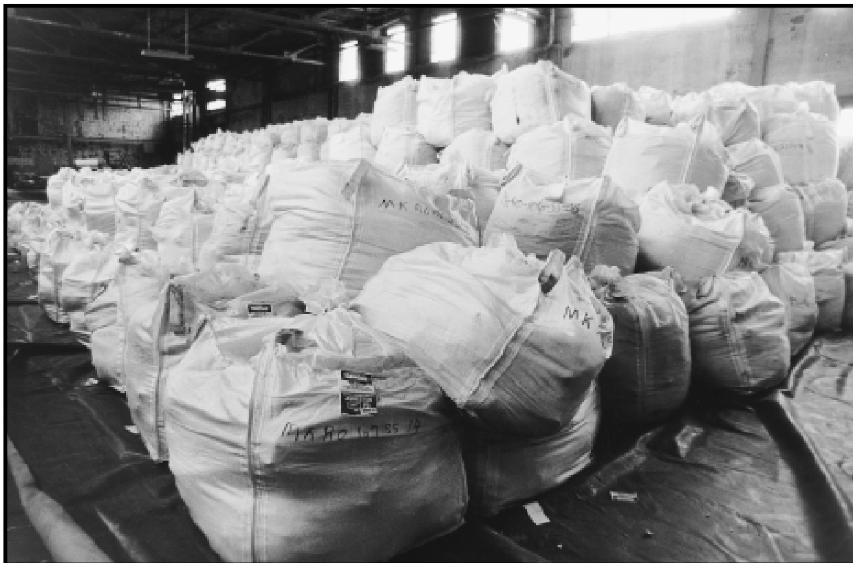
Radioactively-contaminated asbestos removed from buildings that processed uranium for the Manhattan Project. Downtown St. Louis FUSRAP site, Missouri. January 29, 1994.
