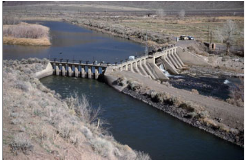
Truckee Canal Headworks and Derby Diversion Dam
