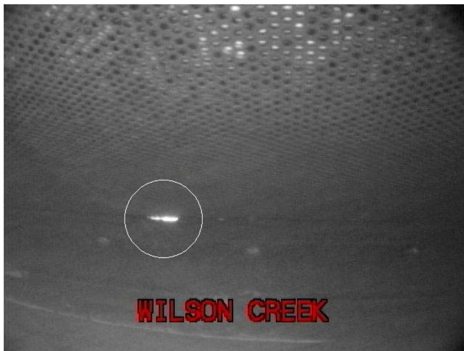
Figure 49. Gap Between the Bottom Seal and the Screen Observed at Wilson Creek in June 2002
