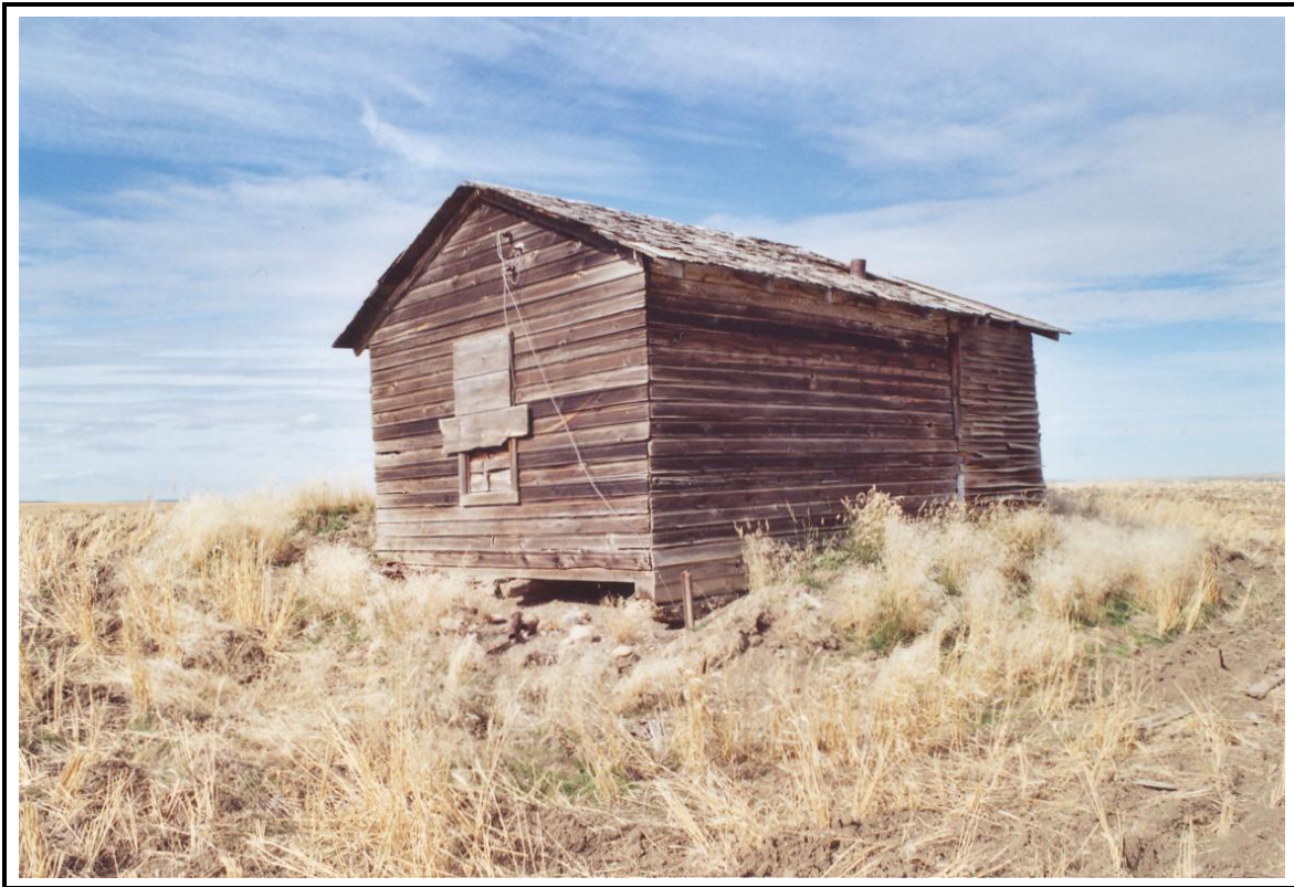
Figure 20. The Feature 1 house at 24CA987. View to the northwest.
