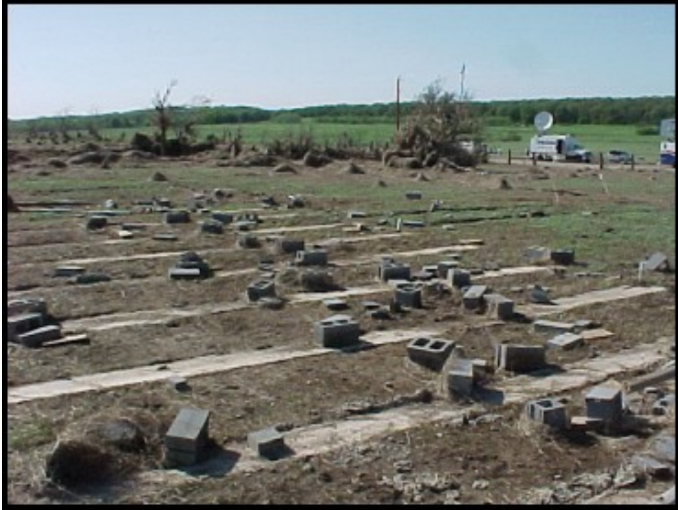
Picture 9: Close-up view of the same destroyed mobile home site as in Picture 8, except looking northwest. The only remnant of the mobile home was the steel beam frame, found approximately 200 yards to the northwest of the original home location. (In the field behind, and to the left of, the television satellite truck in the background of this photograph.) (See Figure 6 for location of picture).
