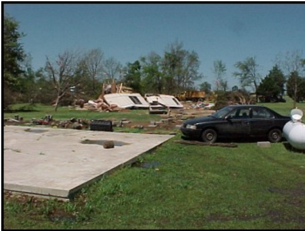
Picture 2: Looking north-northwest. A mobile home was lofted and deposited upside-down about 40 yards from its original location on the blocks just to the left of the automobile. Two injuries requiring hospitalization occurred at this location. Note the vehicle was not moved. (See Figure 5 for location of picture).
