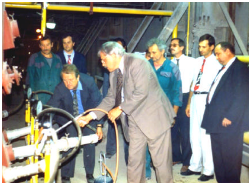
Loren Schulze, USAID/Slovakia, helps inaugurate a kiln at the Tisovec lime factory, 1997. The EAPS Slovakia program helped renovate the kiln and convert it from coke to gas fuel, greatly reducing polluting emissions and improving plant efficiency.
