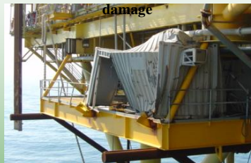
Sub-cellar deck light damage
