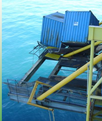
Sub-Cellar North Extension
