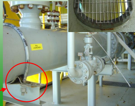
Mica Pig Launcher shifted
