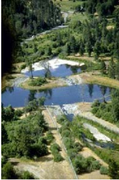
Figure 7. View of Hamilton Ponds on lower Grass Valley Creek. The ponds trap fine sediment, mostly sand and fine gravels derived from decomposed granite. Photo courtesy of the U.S. Bureau of Reclamation.
