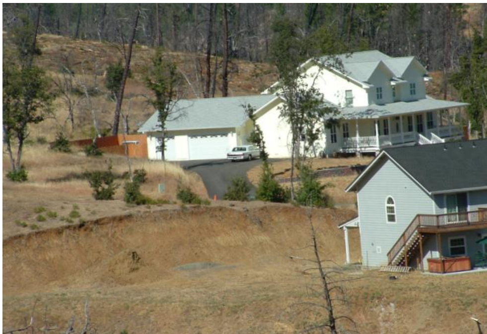
Figure 17. Example of rill erosion on cutbank in new housing development near Weaverville, California.
