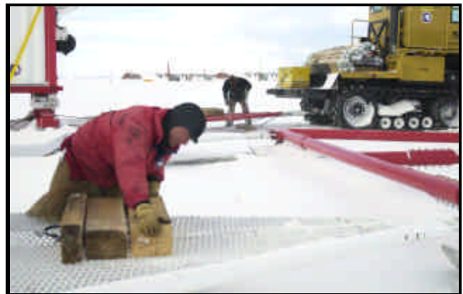
Heavy equipment operator Brad Johnson secures blocks to the tongue of a sled. Behind him is John Penney, who is working on a tractor.
