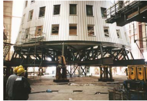
Figure 2 De Bolder on the transition structure
