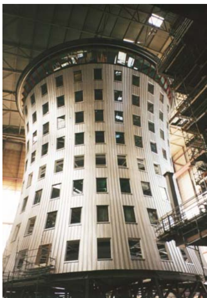
Figure 1 De Bolder under construction in the industrial plant
