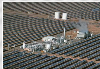
Parabolic Trough Rankine Cycle Power Plant
