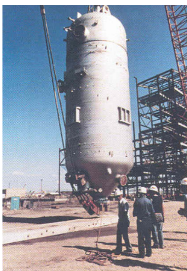
The installation of a Lurgi gasifier
