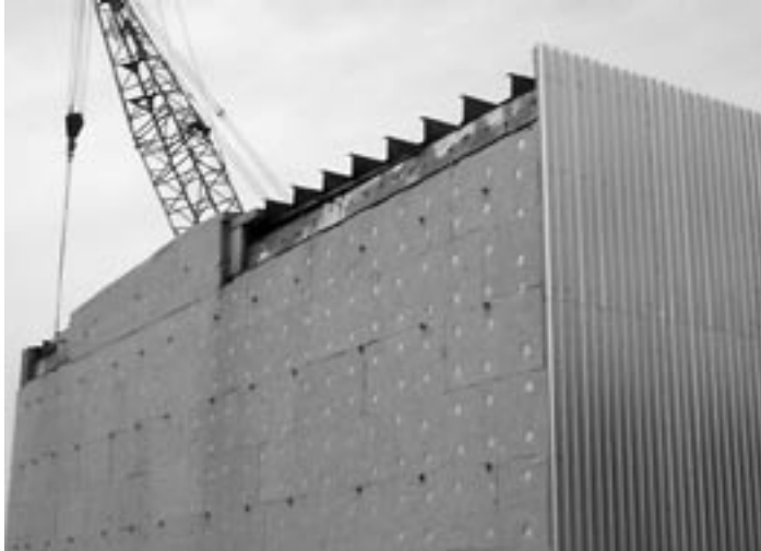
Photo 1. Insulation panels during installation.
