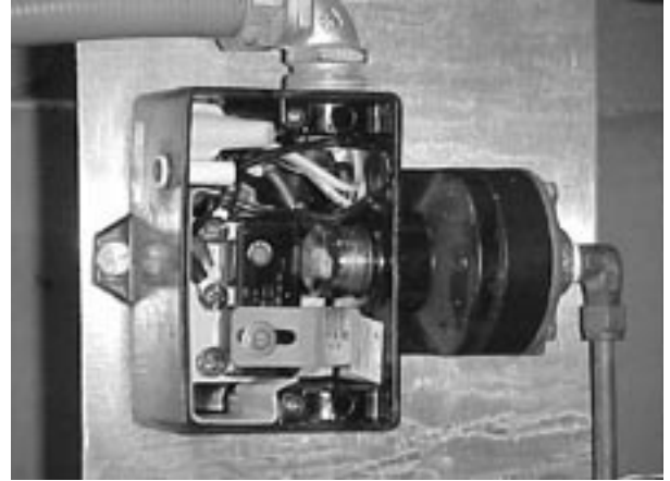
Photo 9. People get creative to defeat safety controls. Here a Popsicle® stick is stuck into an air switch to force it always open.
