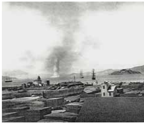
Blasting of Arch Rock in 1901. View from San Francisco. Alcatraz Island is in the right middle ground. Photograph courtesy of U.S. Army Corps of Engineers.
