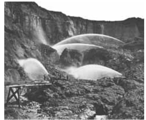
Hydraulic mining at the Malakoff Diggings in the foothills of the Sierra Nevada. Photograph by Carleton E. Watkins , courtesy of the Bancroft Library, University of California, Berkeley.
