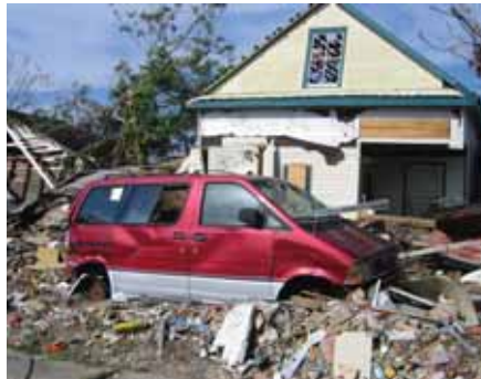
Typical scene of hurricane destruction in the east half of Biloxi, Miss.
