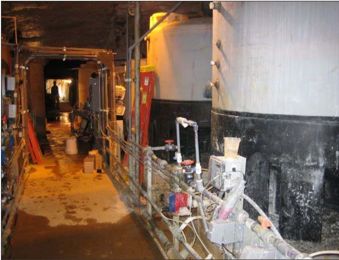
Figure 4. Looking towards the mine entrance.
