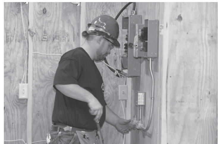
Electricians join the wires in boxes with specially designed connectors.
