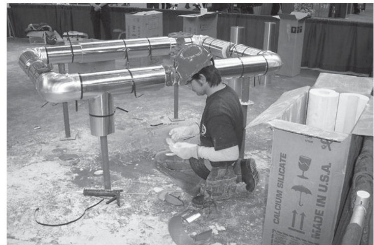
Insulation workers install the materials used to insulate buildings and equipment.
