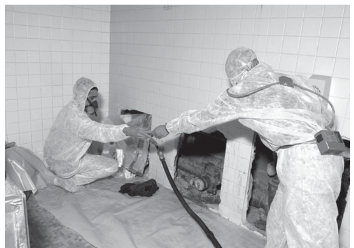
Most hazardous materials removal workers are required to wear respirators to protect them from airborne particles.
