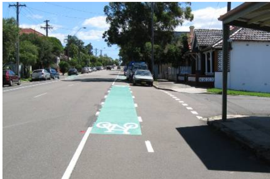
Figure 12. Green-colored pavement used to highlight a bicycle lane as it crosses through an unsignalized intersection in Sydney, Australia.
