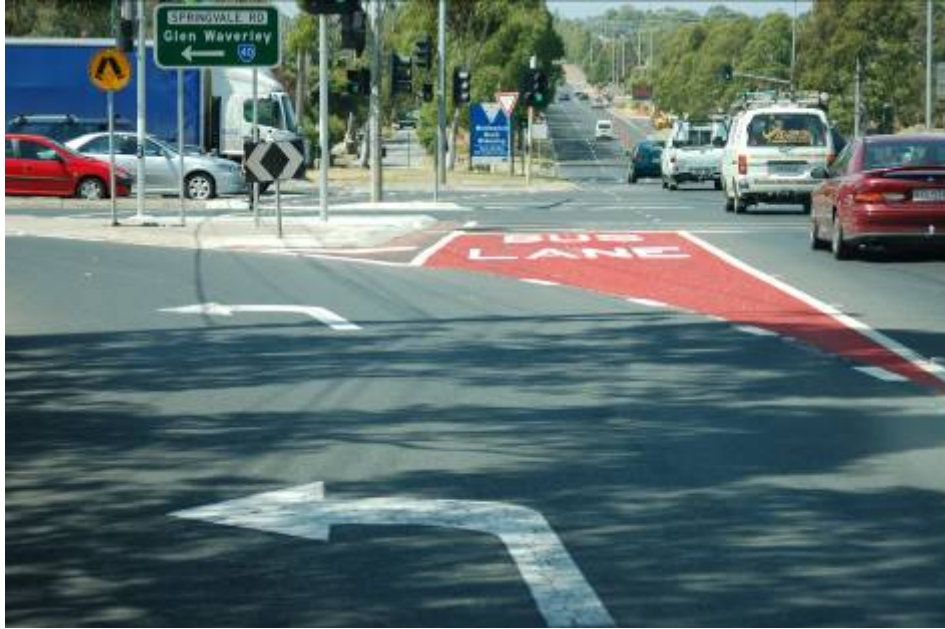
Figure 11. Red-colored pavement used to mark a bus queue-jump lane at a signaled intersection in Melbourne, Australia.
