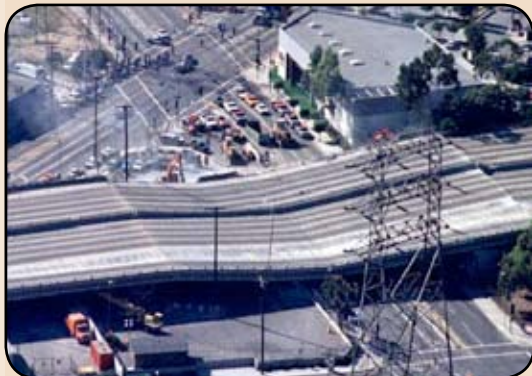
Part of Interstate 10 west of downtown Los Angeles collapsed in the shaking of the 1994 Northridge earthquake.
