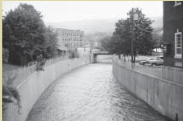
Adams’s 2.2-mile-long flood-control system includes this 1.2-mile paved concrete chute, along with other sections having earth or gravel channels with concrete walls or riprapping. Water flowing through the structures is spread out over an unnaturally wide, shallow channel with little or no shading. “The summer sun just bakes the water,” says HooRWA Executive Director Lauren Stevens.
