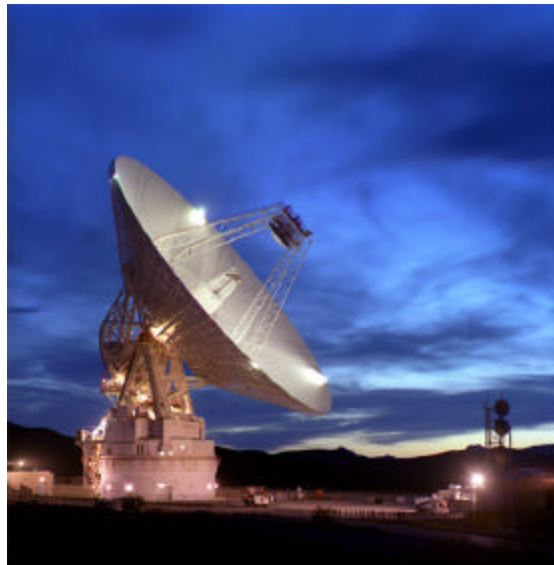
Figure 2: 70-Meter Deep Space Communication Antenna
