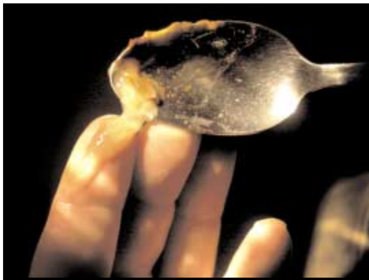
A sample of slime scraped from the water plant pipes turns out to be a mixture of pteropod remains and bacteria. Similar goo has clogged the filters.
