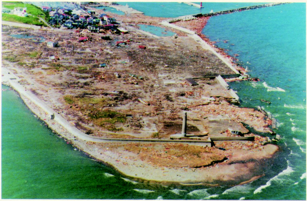
Figure 1: A view of tsunami damage from the south of Aonae, a small town on Okushiri, an island in the Sea of Japan (courtesy of Y. Tsuji).
