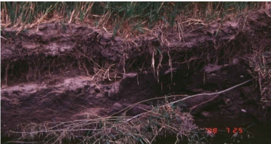
Figure I-1.—Weak soil developed on reservoir-related sediment at the mouth of Canyon Creek.
