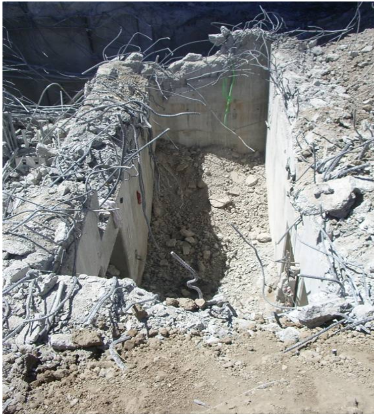
Figure B-22. ECCS B210 area stairway ready for backfill.
