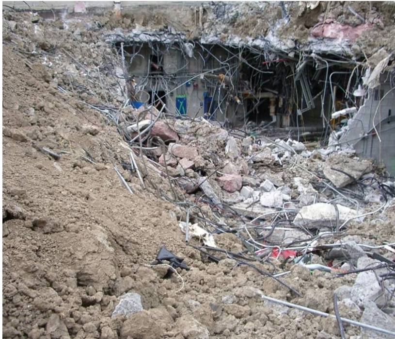
Figure B-6. B203 Area ready for backfill.
