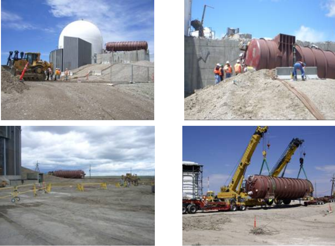
Figure 14. Remove borated tank from TAN-650 top level.
