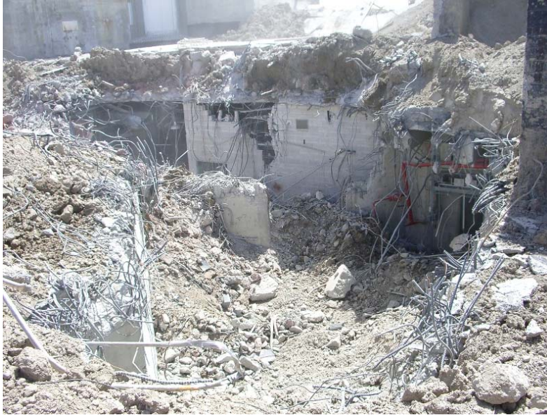
Figure B-3. B105A/B209 Area ready for partial backfill.
