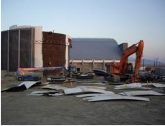
Figure 21. Process, segregate and package CV material for disposal and dispose.
