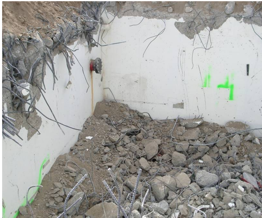
Figure B-10. B104 Area ready for backfill.
