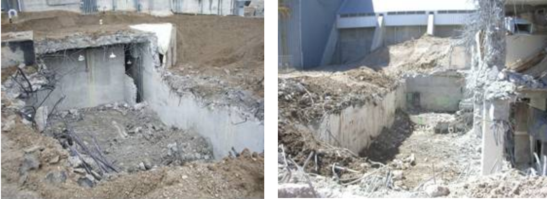
Figure 5. Process TAN-630 structure to three feet before grade.
