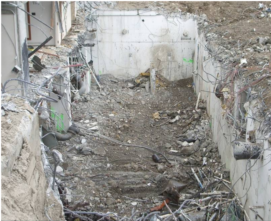
Figure B-12, B103 east area ready for backfill.
