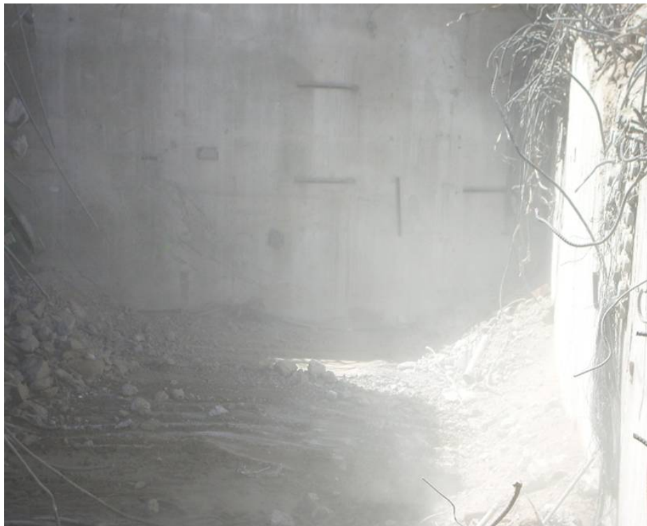
Figure B-16. North portion of B101 area ready for backfill.
