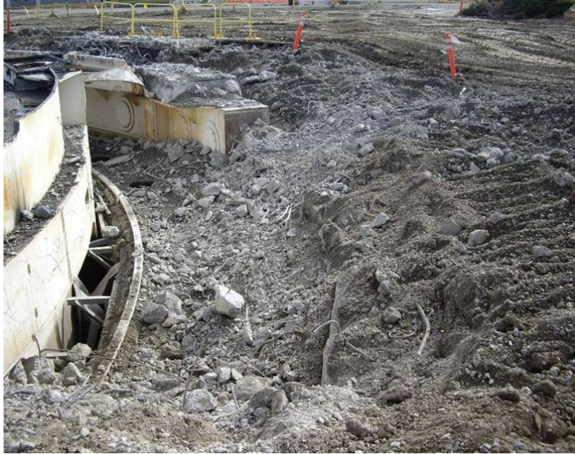
Figure B-23. B229 Area ready for backfill.
