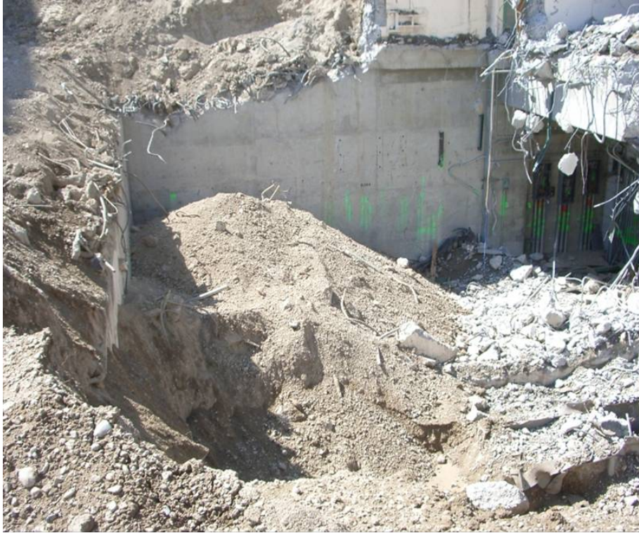
Figure B-19. West portion of B103 and B102 area ready for partial backfill.
