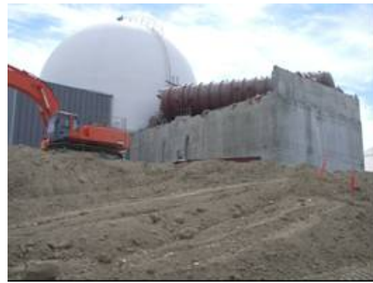
Figure 13. Remove roof, north and east cinder block walls top level to access borated water tank.
