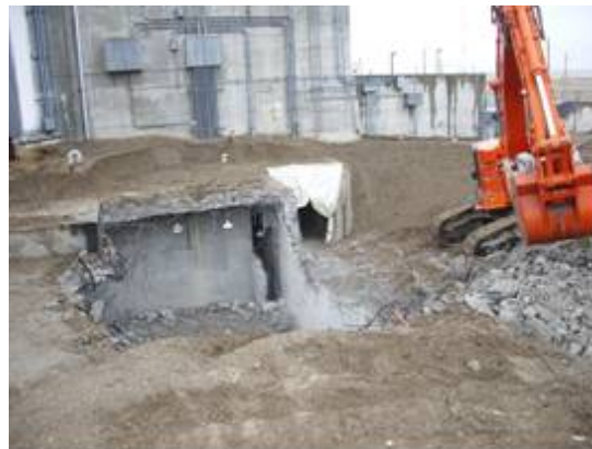
Figure 1. Remove shielding soil from TAN-630, TAN-650, and Room 219 and stage.
