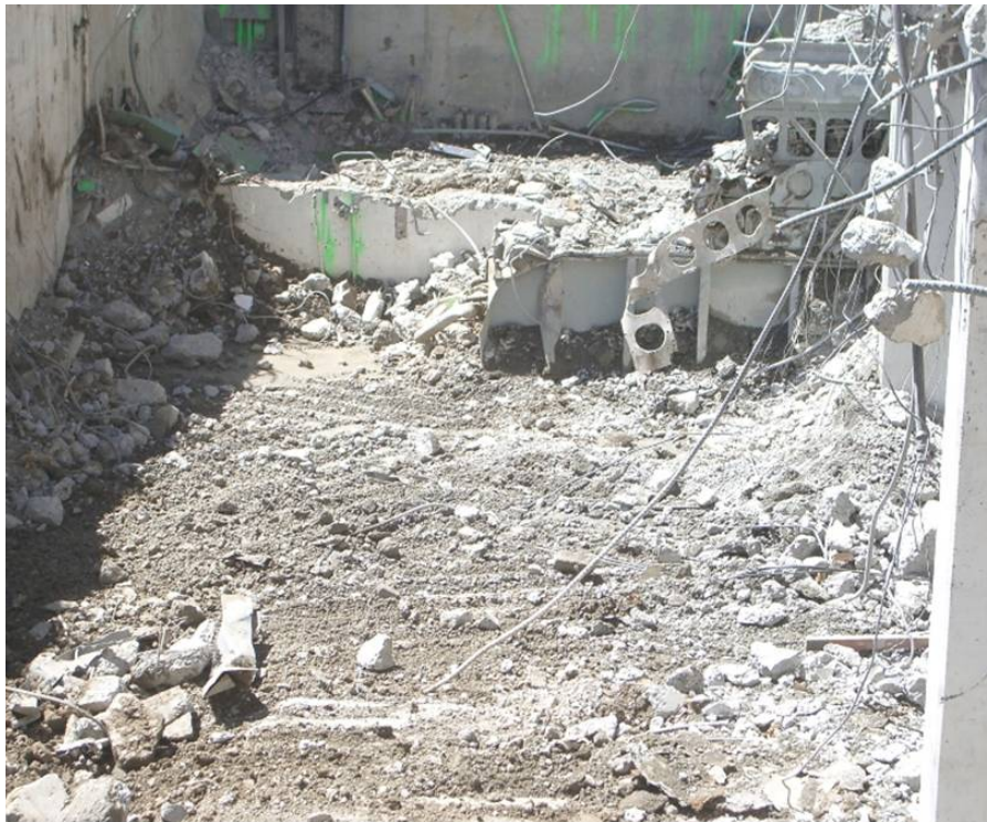
Figure B-18. Evidence of Segmented Diesel Generator Removal from TAN-630.
