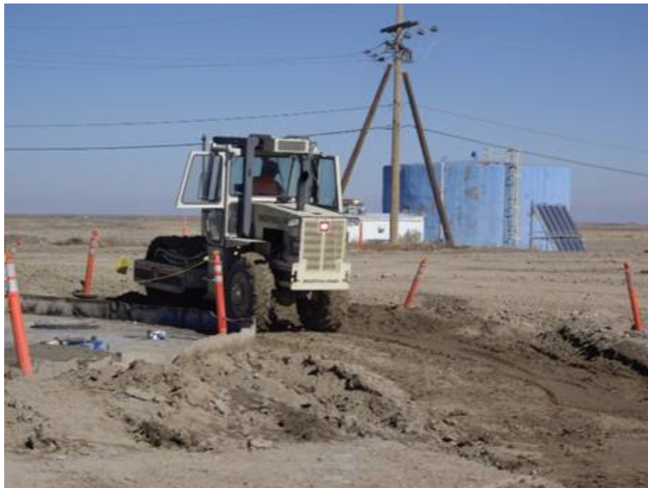
Figure 22. Backfill remaining areas to grade.
