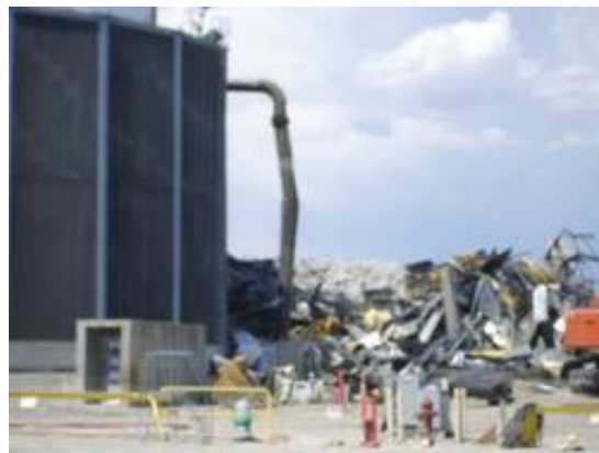
Figure 3. Remove boilers, and generator, borated water tank, and other large equipment.
