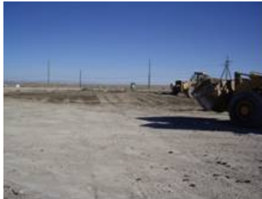
Figure 23. Construct final cover over CV area.
