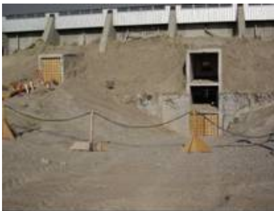
Figure 9. Remove equipment and piping.
