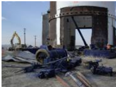
Figure 17. Remove Containment Vessel Dome and remove polar crane.
