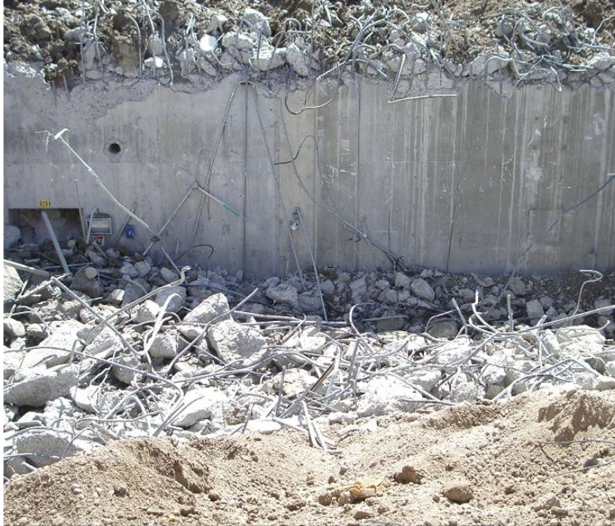
Figure B-9. B203 Area ready for backfill from South and North.
