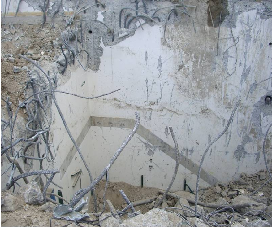
Figure B-7. B203/B201/B204/B205 Areas ready for backfill.
