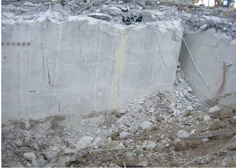
Figure B-1. B219 areas ready for backfill.
