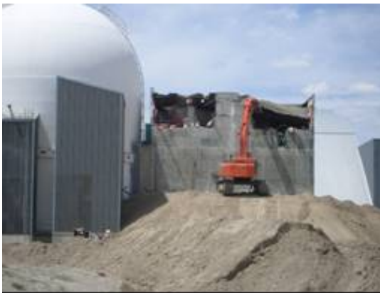
Figure 13. Remove roof, north and east cinder block walls top level to access borated water tank.
