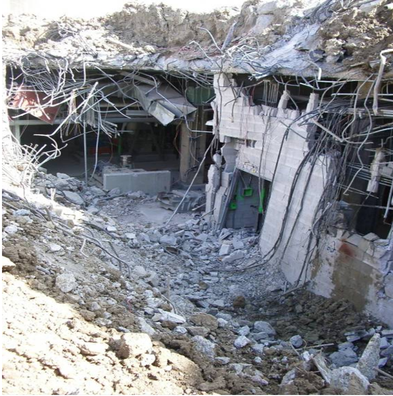
Figure B-5. B202 Area ready for backfill.
