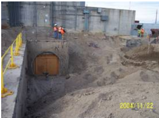
Figure 2. Build access road to tunnel on east side of TAN-650.
