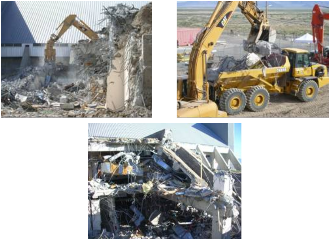
Figure 15. Process, package and dispose remaining structure, equipment, and piping.
