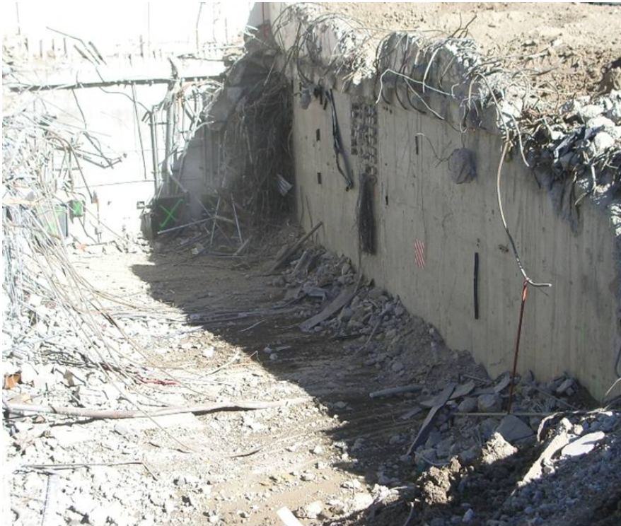
Figure B-14. North portion of B101 area ready for partial backfill.
