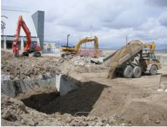
Figure 7. Backfill areas to proper grade as needed.
