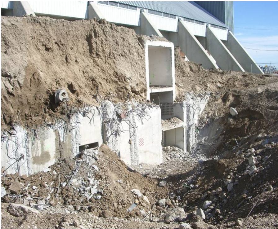
Figure B-20. West portion of TAN-630 area ready for partial backfill.
