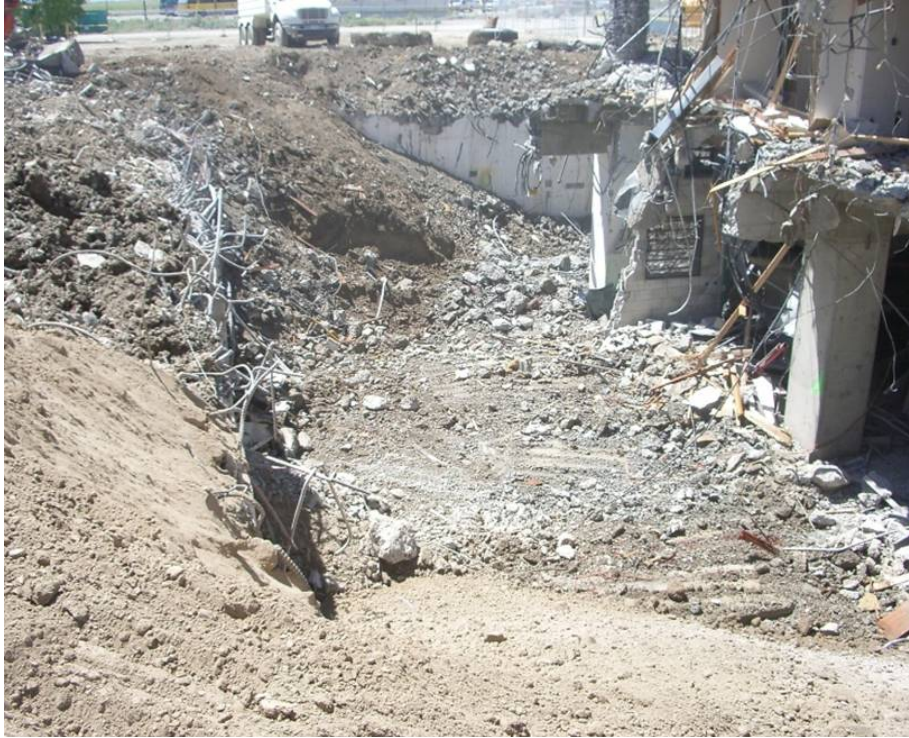
Figure B-15. East portion of B101 area ready for backfill.
