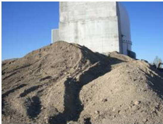
Figure 8. Construct soil ramp to access upper structure.
