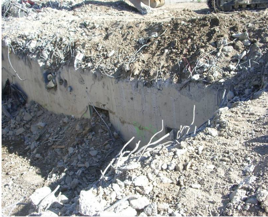
Figure B-13. NE portion of B101 area ready for backfill.
