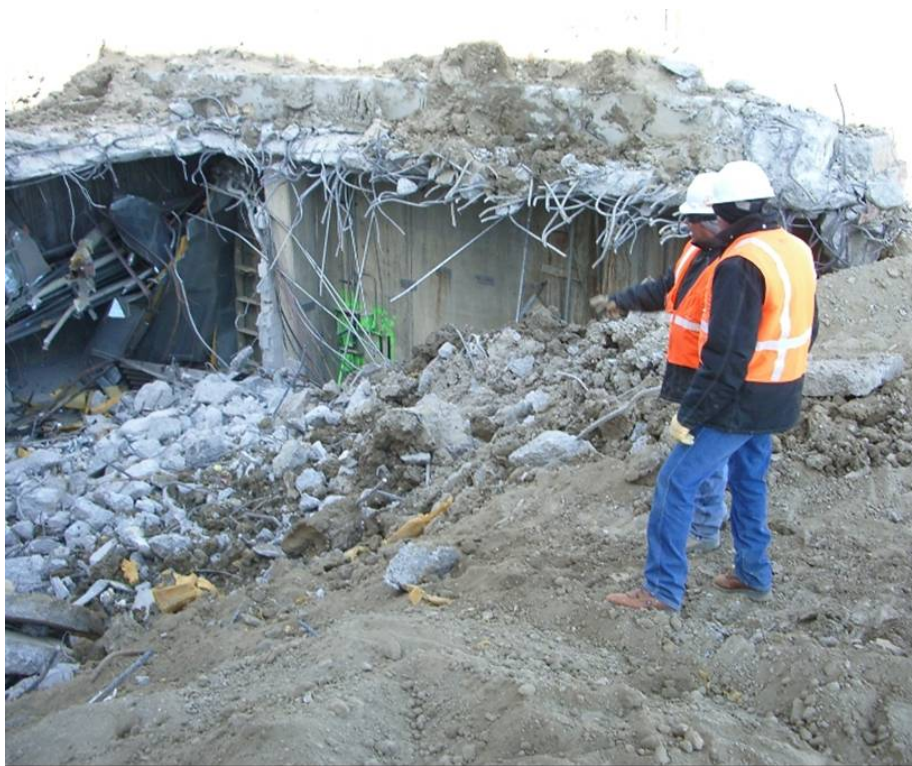
Figure B-8. B203 Area ready for additional backfill.
