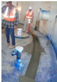
Figure 11. Fill lower CV, and sumps with inert material.
