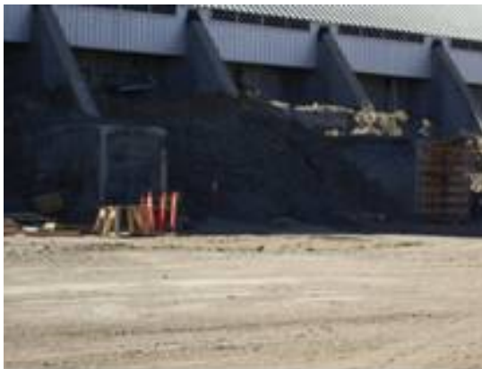
Figure 10. Complete SMC tunnel opening closures.
