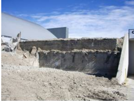
Figure 1. Remove shielding soil from TAN-630, TAN-650, and Room 219 and stage.
