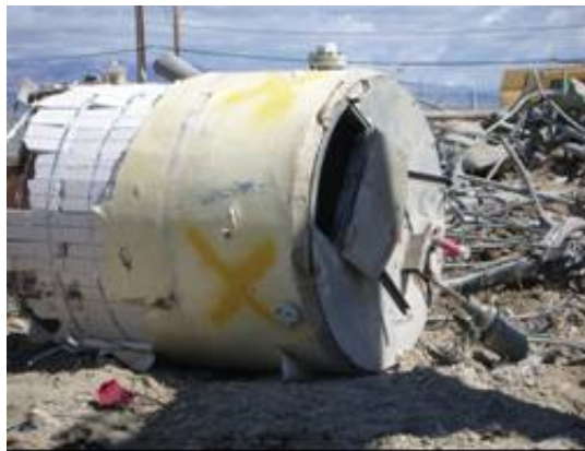
Figure 3. Remove boilers, and generator, borated water tank, and other large equipment.
