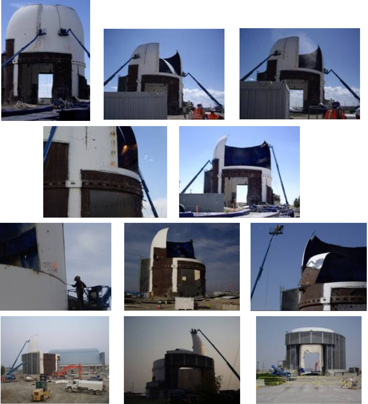
Figure 18. Demolish Containment Vessel.
