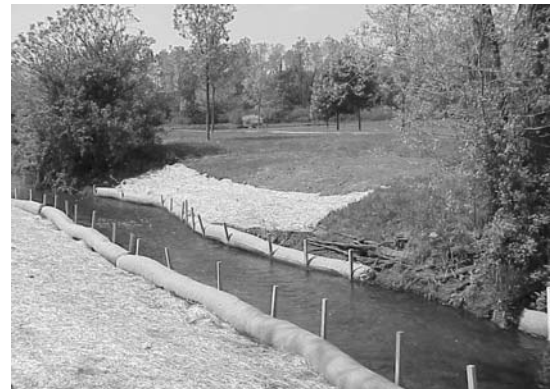
Firefighters Park Streambank Stabilization After
