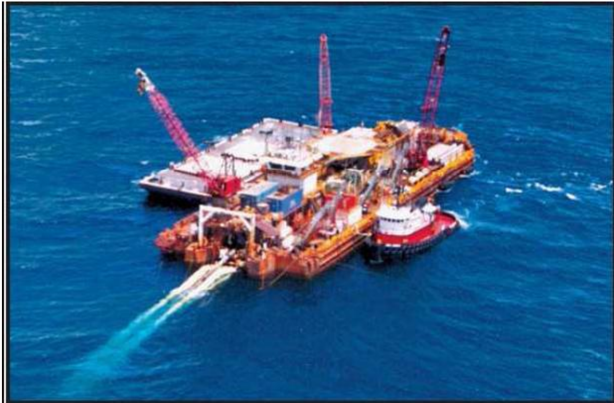
Figure 24-3 Representative Pipelaying Barge and Support Vessel
