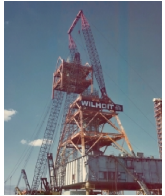
As part of Shuttle program modifications to Apollo era facilities, a launch umbilical tower, above, is detached from the Mobile Launcher to be transported, at left, to Launch Pad 39A.
