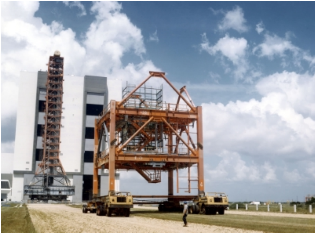
As part of Shuttle program modifications to Apollo era facilities, a launch umbilical tower, above, is detached from the Mobile Launcher to be transported, at left, to Launch Pad 39A.
