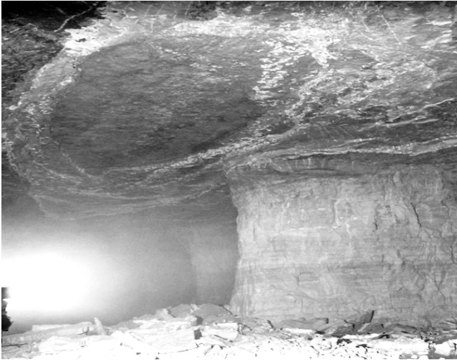
Figure 1. Typical oval shaped roof fall associated with horizontal stress in the roof.
