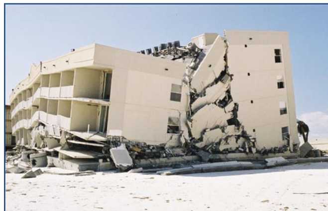
Figure 1. Poorly sited building on shallow foundation undermined by erosion.
