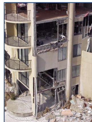
Figure 1. Poorly sited building on shallow foundation undermined by erosion.
