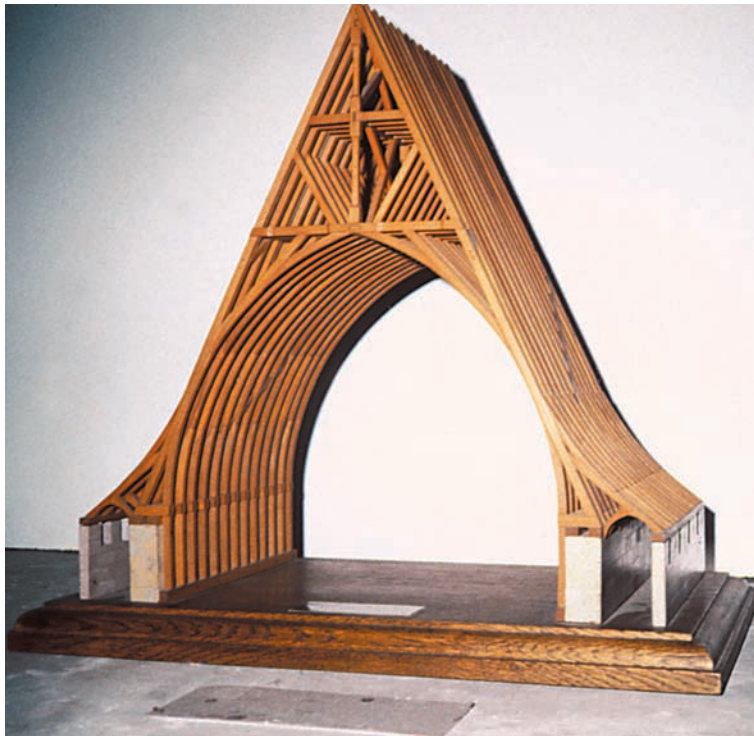
Fig. 6. Deneux's model (CRMH, Paris) of the roof of the upper hall of the Château de Sully-sur-Loire, 1401-1460. Framing is of uniform scantling, in the northern European tradition, and closely spaced.
