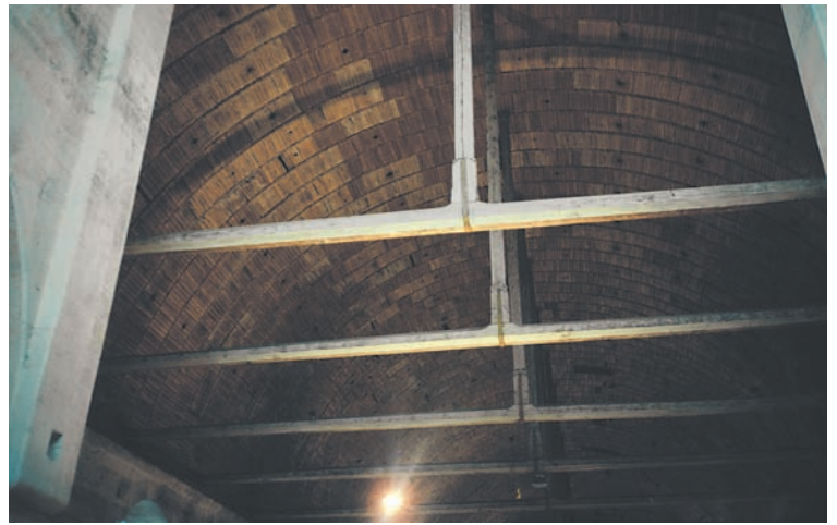
Fig. 17. Tonnerre, kingpost and tie beam assembly with vault paneling (some restored). Each panel spans about 26 in. of the vault surface.
