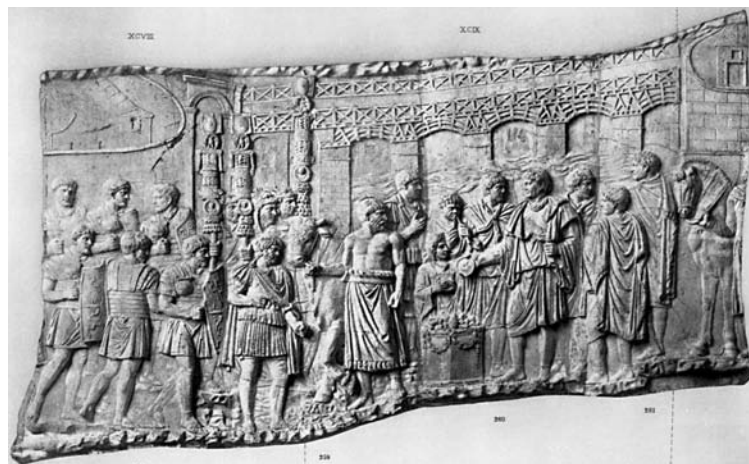
C. Chicorius, 1904 Panel from Trajan's column depicting Apollodorus's bridge (ca. 105) across the Danube. Trussed segmental arches spring from triangulated supports to carry the bridge deck. Triangulated railings may help.
