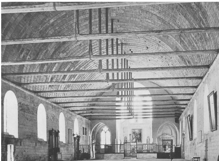
Fig. 14. The open ward of the Maison Dieu, with clear span and height to top of vault both about 60 ft.; design is based on equilateral triangle.
