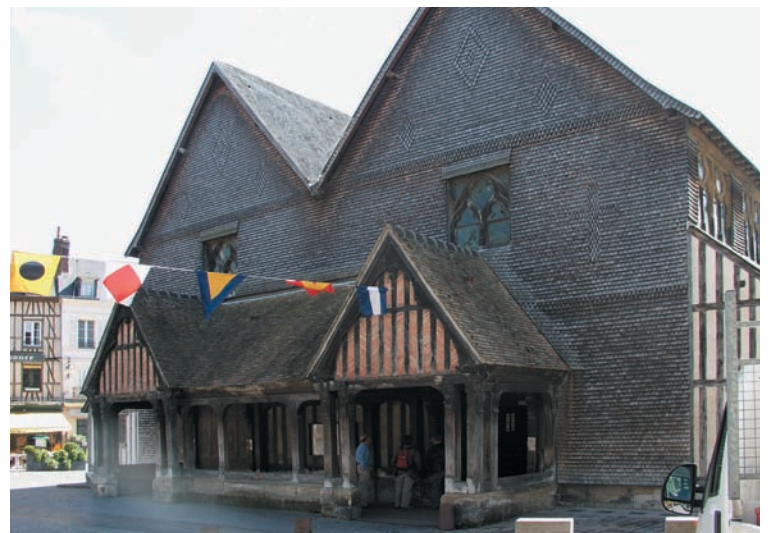
Fig. 11. Twin porches and double nave at Ste. Catherine's. Exposed colombage visible at right on lean-to addition and porch pediment.
