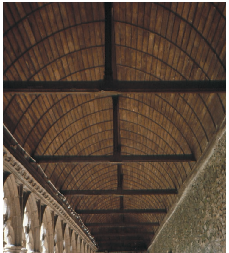
Fig. 4. Fifteenth-century cloister vaults at Tréguier Cathedral in Brittany, illustrating typical charpente lambrissée with intermediate kingpost trusses.
