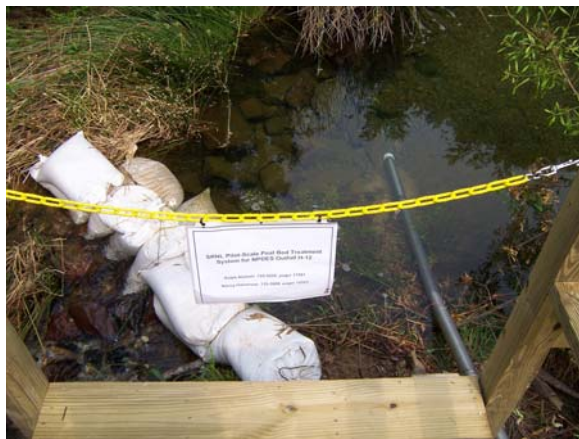
Figure 8. Sand bag dam and influent pipe casing
