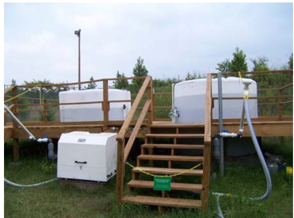
Figure 7. Access deck – Tank 1 on the right and Tank 2 on the left
