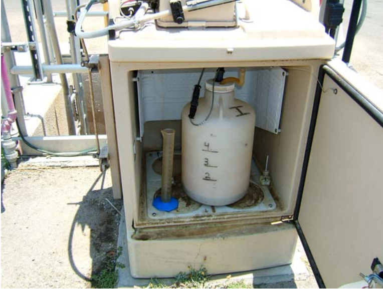
Influent Sampler Composite Bottle
