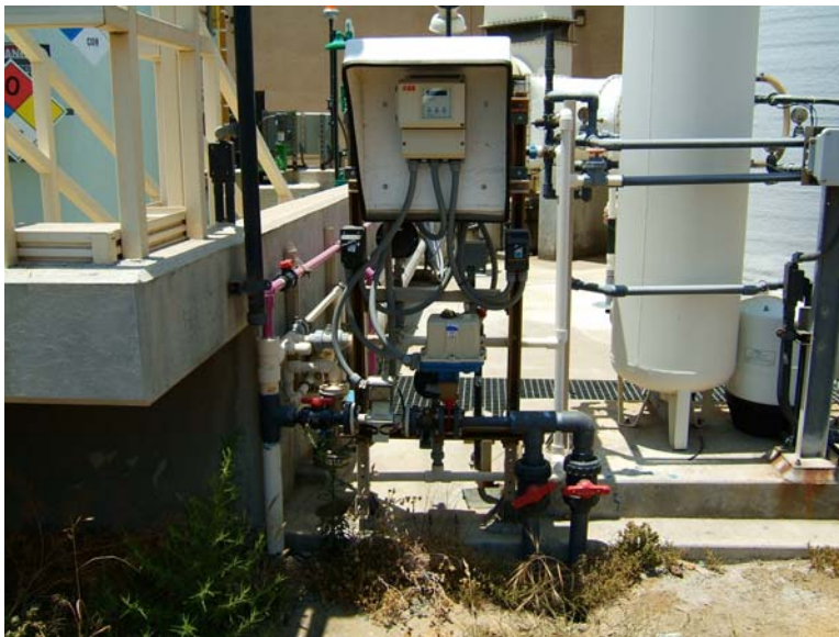
Ferric Chloride Dilution System for JB1
