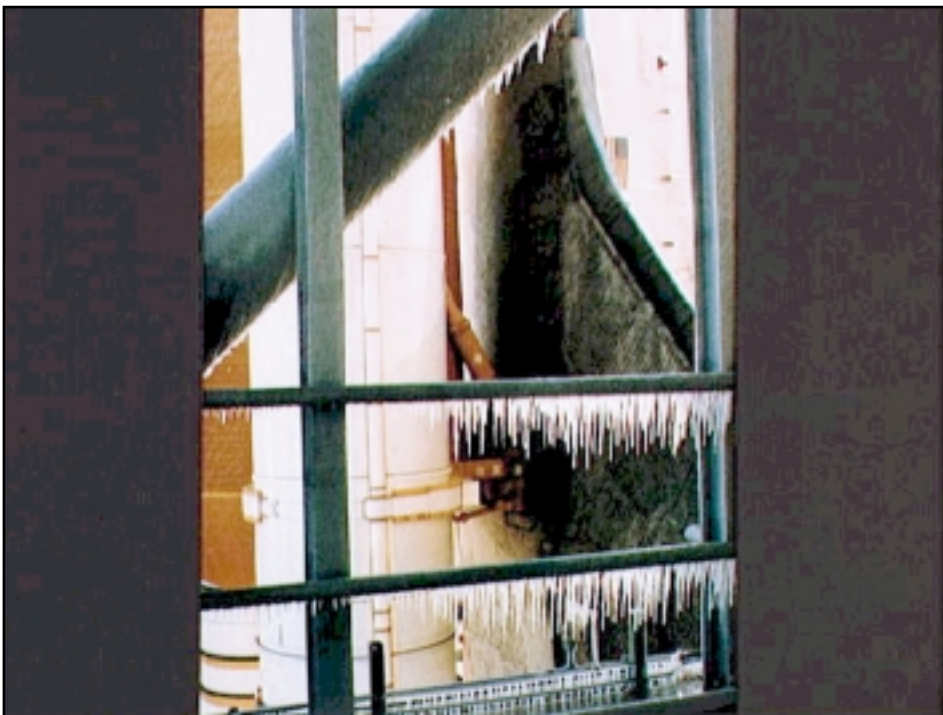
Icicles on the launch pad show the temperature the morning of the Challenger's launch.
