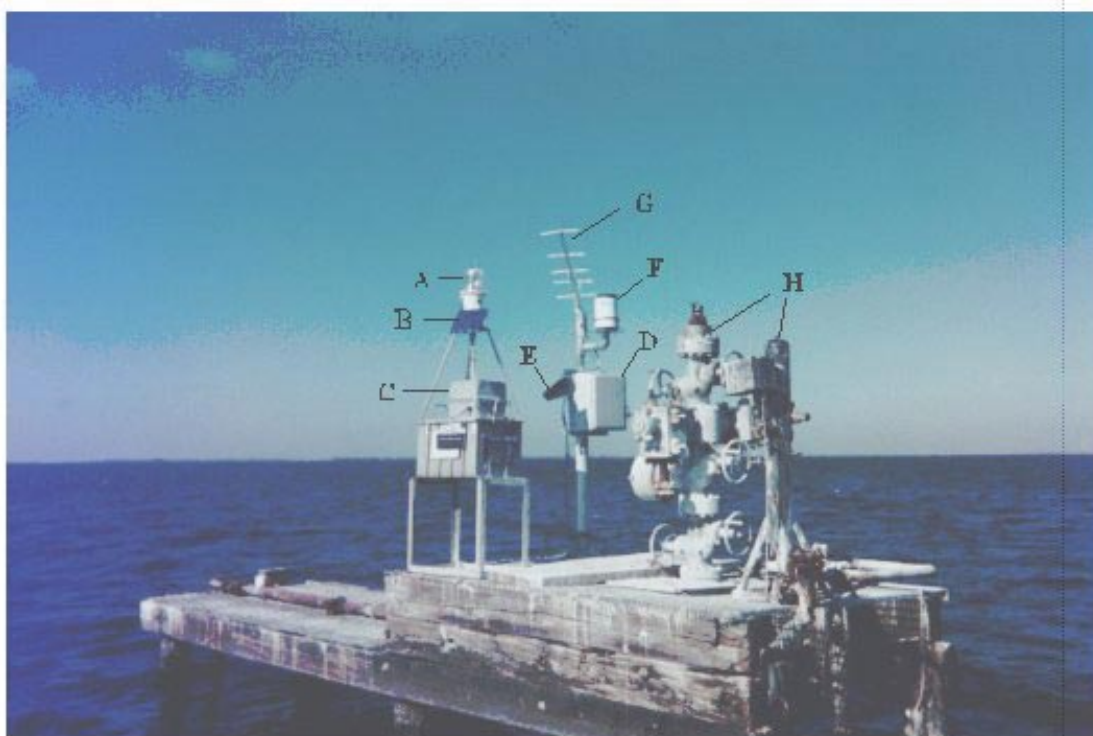
Figure 3.4. Picture of the sampling system platform taken during the January 9, 2001 site visit.
