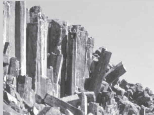
Exhibit H: Columns of basalt showing their tendency to fall down steep slopes. (Photo: National Park Service)
