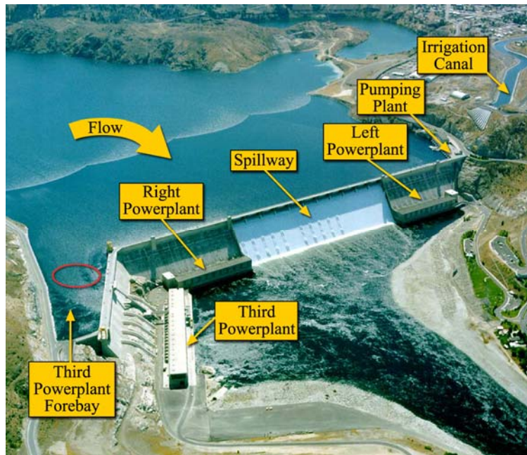
Figure 2.2. Study Site Location (red) Near Third Powerplant, Grand Coulee Dam in 2001 through 2004
