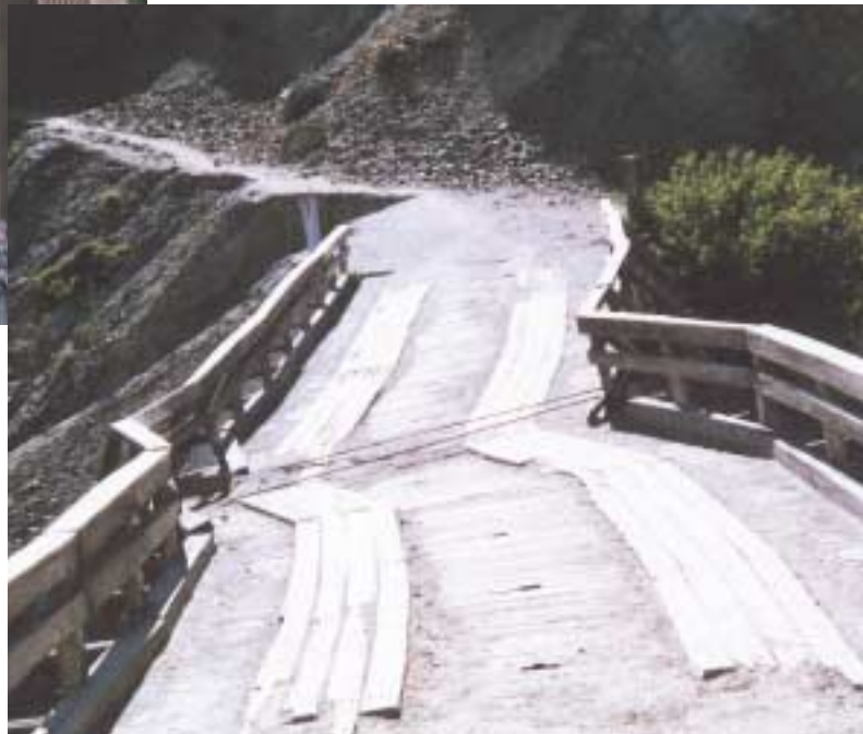
Very few roads are paved in Bolivia, and landslides can make travel difficult and occasionally hazardous.
