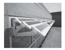
Figure 3-34. Photo of PV panels integrated into sun-shading system. Photo courtesy of Kawneer Company; Photo: Gordon Schenck, Jr.
