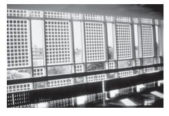
Figure 3-33. Photovoltaics integrated with glazing. In this type of application, the solar cells provide shading and generate electricity. Photo courtesy of DOE/NREL; Photo: Paul Maycock
