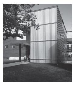
Figure 3-27. Exterior view of Rapson Hall at the University of Minnesota using channel glass with translucent insulation. Architect: Steven Holl Architects; Photo: Warren Bruland
