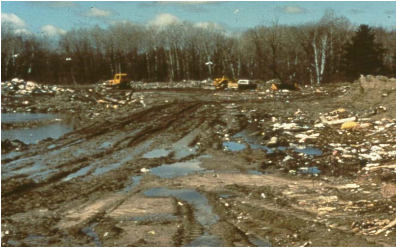
Photo 1. Landfill where storm water has been allowed to pond; SWANA MOLO 2004. (Ref. 4)
