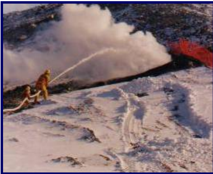
Photo 13. Firefighting at the Exit C&D landfill Ohio (Landfill Fire Conference, Ohio 2006, Ref. 17)
