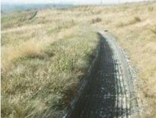
Photo 2. Direct runoff ditch at a landfill, (SWANA, MOLO 2004, Ref. 4).
