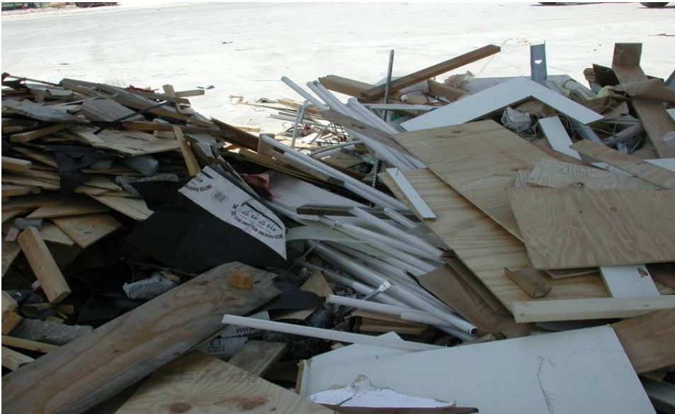
Photo 17. Improper Disposal of Fluorescent Lamps, Townsend 2004 (Ref. 28).
