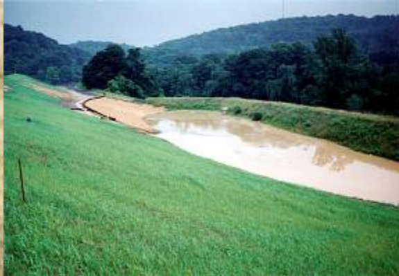
Photo 3. Sediment basin at a landfill, (SWANA, MOLO 2004, Ref. 4).
