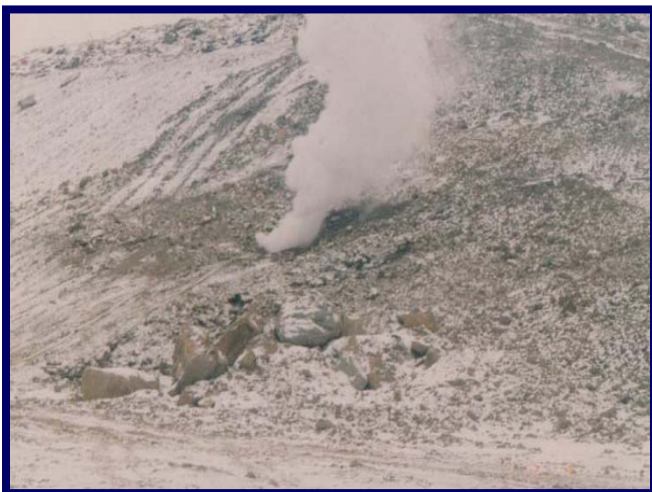
Photo 12. Smoke venting from subsurface fire in 2003, Exit C&D landfill 1 (Landfill Fire Conference, Ohio EPA 2006, Ref. 17)
