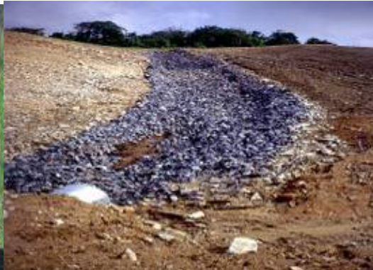
Photo 6, Ditch Lined with Rip/Rap. (SWANA, MOLO 2004, Ref. 4)
