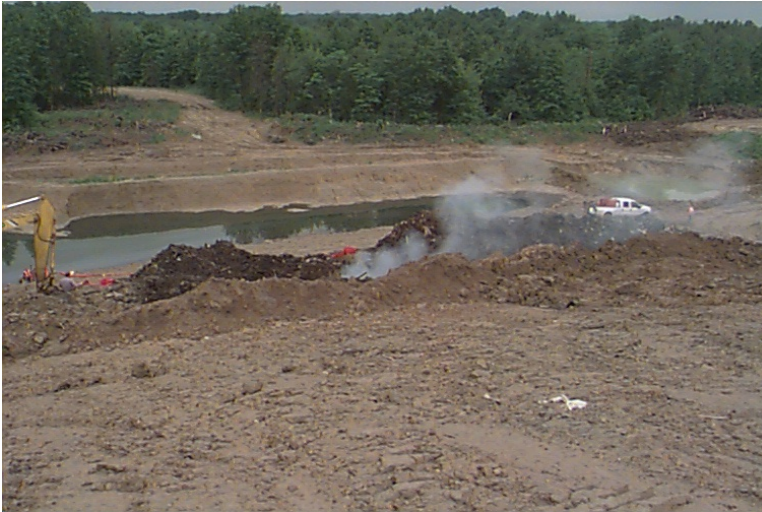
Photo 8. Subsurface landfill fire, Warren Recycling (C&D) Landfill, Ruesch USEPA 2004
