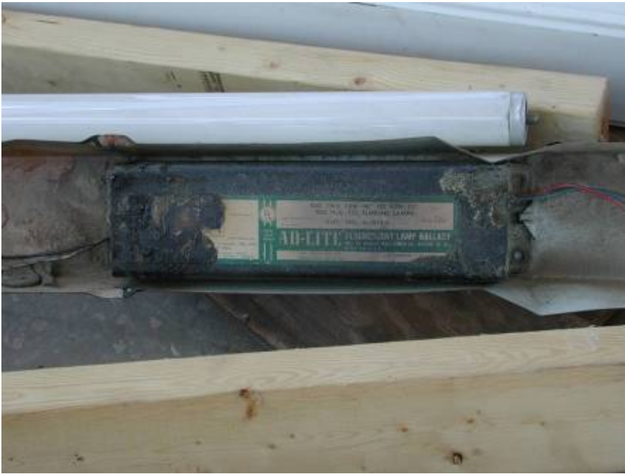
Photo 15. Example of a PCB containing Fluorescent Light Ballast, Townsend 2004 (Ref. 28)
