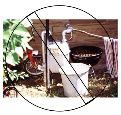
An example of a galvanic corrosion cell. The tenants of this building have "shorted" out this meter by storing metallic objects on the meter set. Never allow customers or tenants to store material on or near a meter installation.
