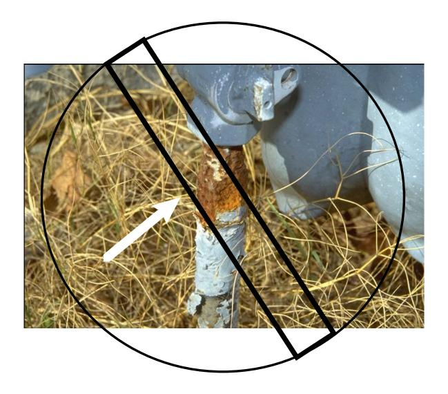
Atmospheric corrosion at a meter riser, as shown above, can be prevented by either jacketing the exposed pipe or by keeping it properly painted. Corrosion is usually more severe at the point where the pipe comes out of the ground.
