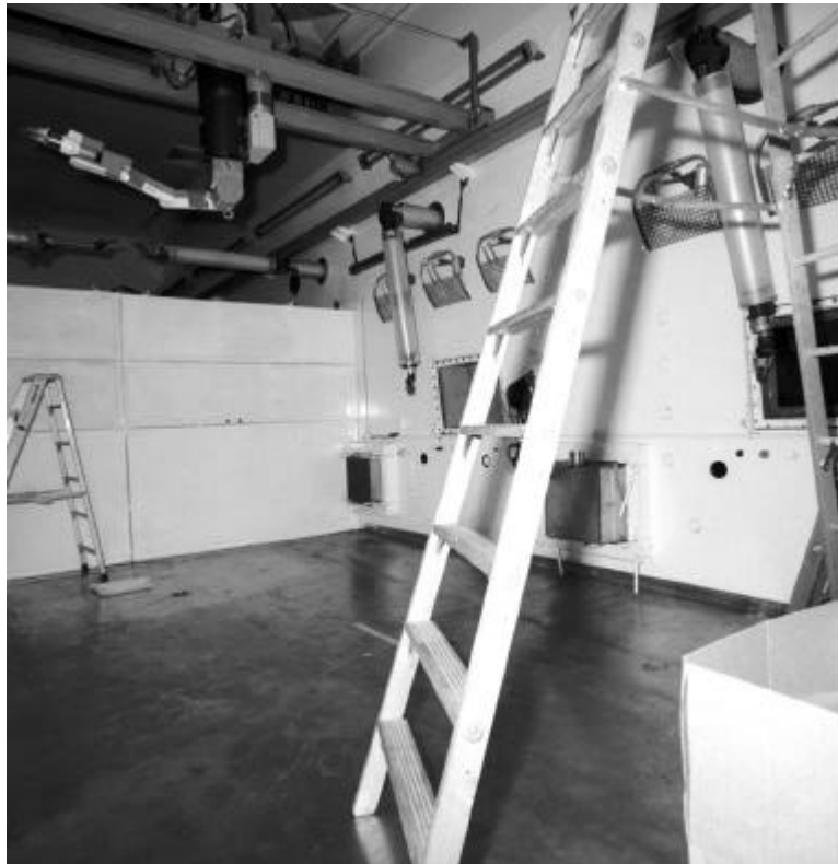
Figure A-9 South Cell View (Interior)
