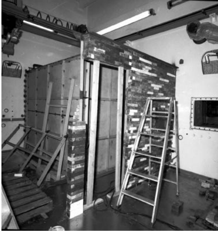
Figure A-8 Compartment 2 Under Construction (Interior)
