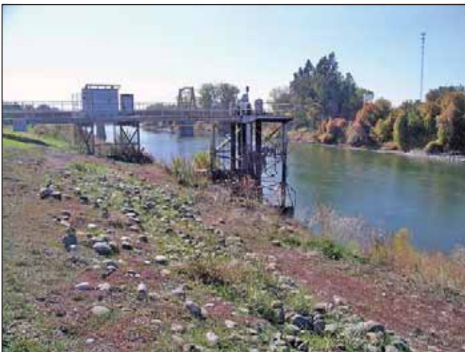
PHOTO 6 – Existing Meridian Diversion.
