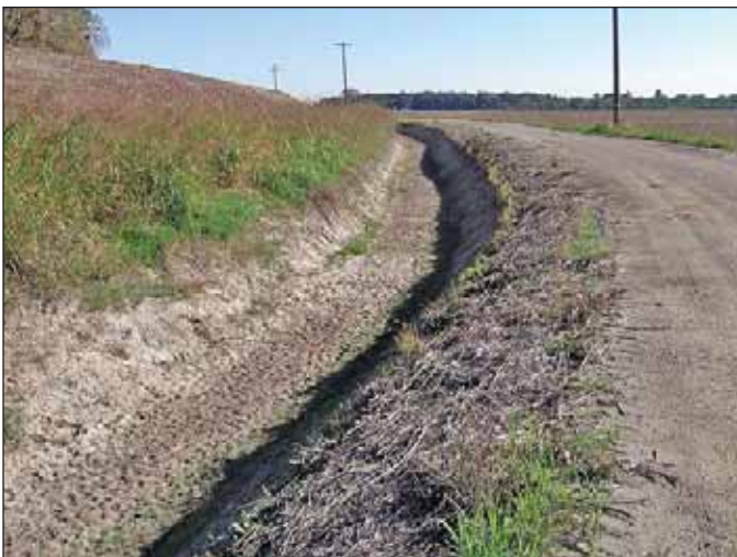
PHOTO 9 – Water Delivery Ditch.
