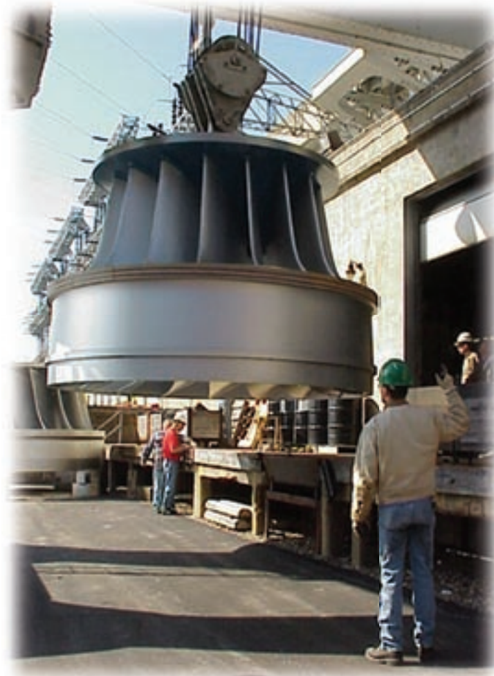
Workers lower a new hydropower turbine to be installed as part of the Osage Project at the Bagnell Dam on Missouri's Lake of the Ozarks.
