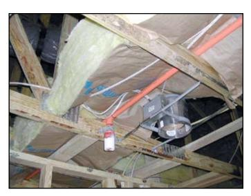
In this illustration, it also is interesting to note that the light fixture appears to be in direct contact with the Kraft paper backing. One might consider this as a potential fire hazard due to the heat emitted from the lamp. This particular fixture, though, is a Type IC rated fixture, and is Underwriters Laboratories (UL) listed for use in direct contact with thermal insulation.
