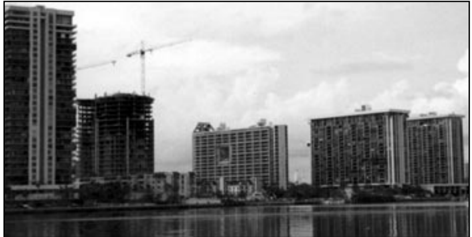
Waterfront condos near completion. (Photo by Rodney Cross, NFIP Bureau)
