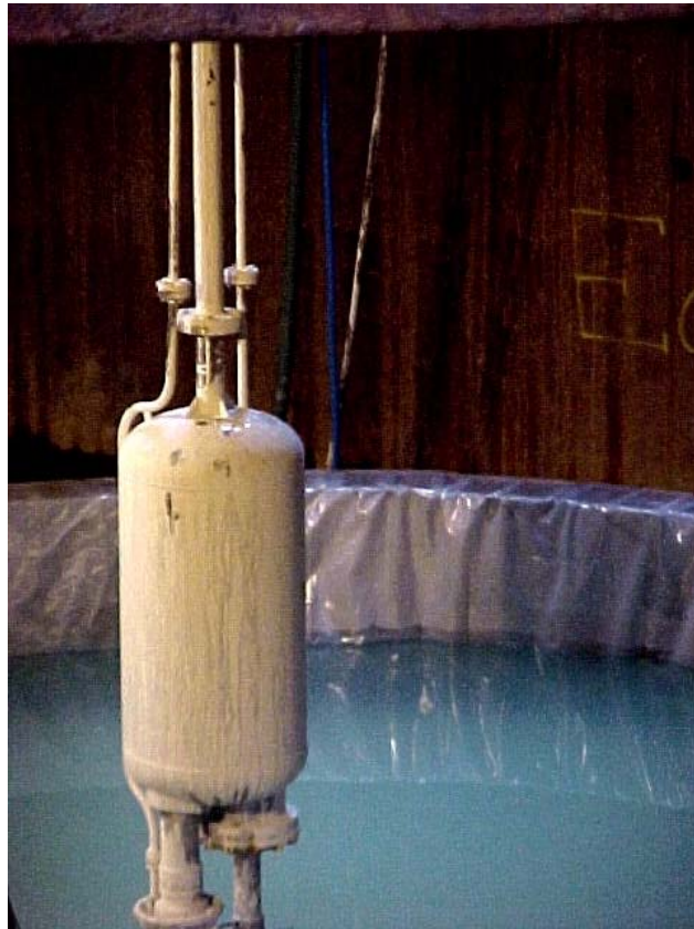
Fig. 14. View of waste simulant on the PMP PV at the TTCTF.
