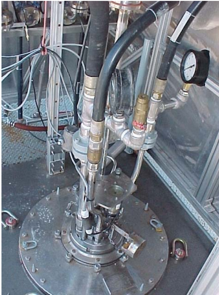
Fig. 7. View of the top of the PMP and drive table inside the TRI.
