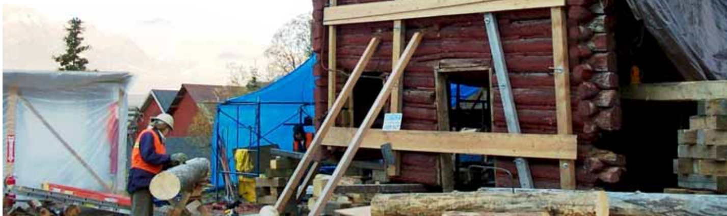
Crews work to stabilize Kennecott's oldest structure, the General Manager's Office
